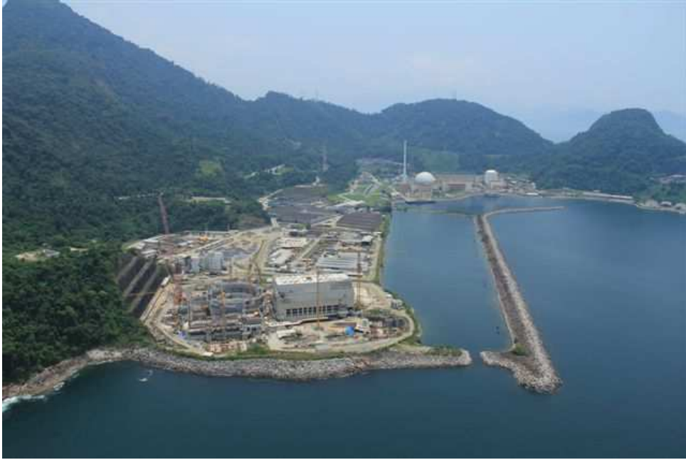
As usinas de Angra 1, 2 e 3
