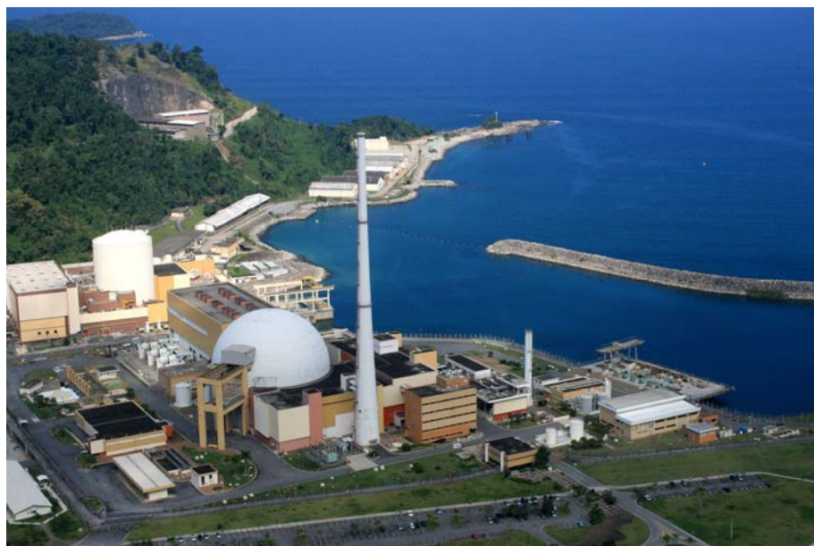
As usinas de Angra 1 e 2
