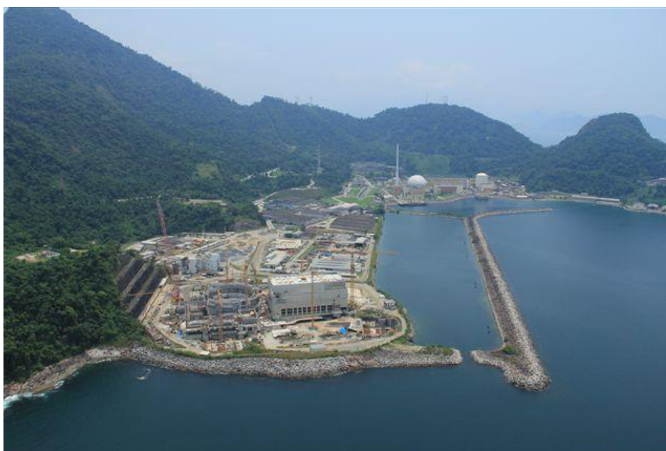
As usinas de Angra 1, 2 e 3
