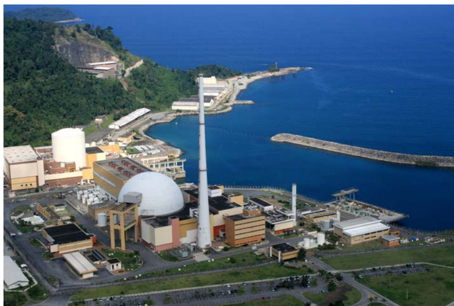
As usinas de Angra 1 e 2
