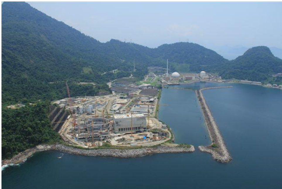
As usinas de Angra 1, 2 e 3
